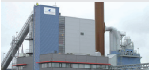
Kemin Energia: Halton industrial central vacuum cleaning system
